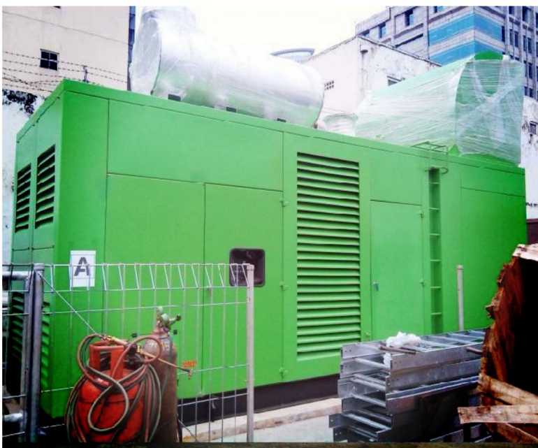
2 Unit MTU 1500 kVA Project Bank Indonesia
