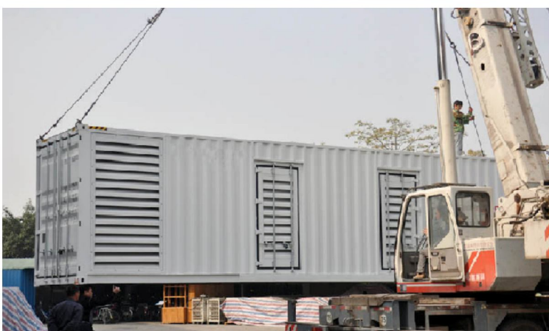
Mitsubishi 1500 kVA Containerized ISO Standard – Project Cargill
